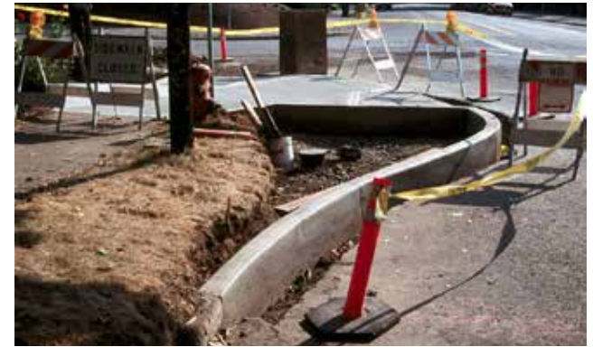
Constructing a Curb Extension, www.pedbikeimages.org/ Dan Burden
