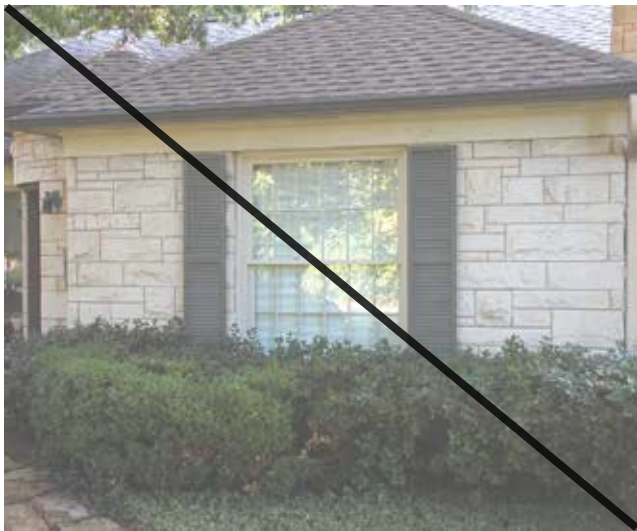
+ Shutters are clearly not sized for the window.
