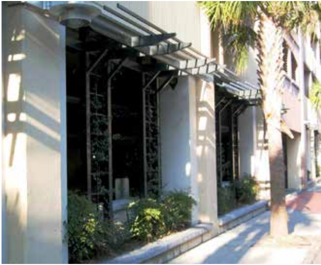
+ MODERN EXPRESSION. Metal arbors - not traditional awnings - can help add ornamentation to buildings as banal as parking garages.
