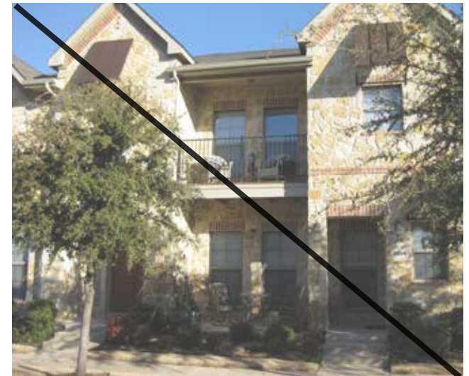
+ Casings do not meet the 3 1/2” requirement.
